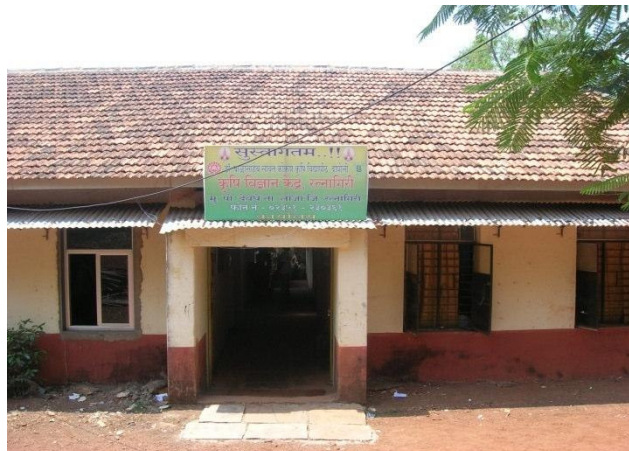
Administrative Building of KVK, Lanja (Ratnagiri)
